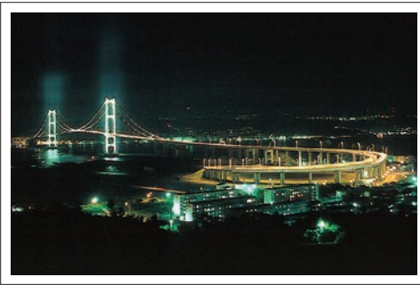
Hakucho Bridge Muroran
