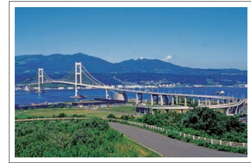
Hakucho Bridge Muroran
