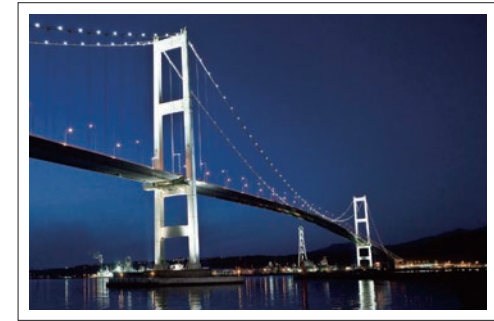
Hakucho Bridge Muroran
